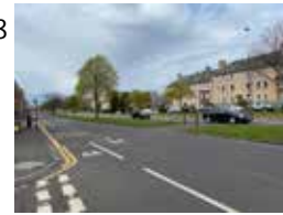
Craigroyston Community Centre
